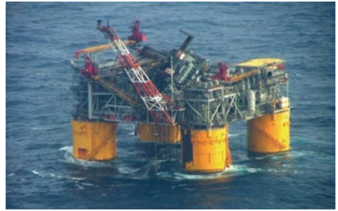
Widespread platform damage in 2005 led to a reassessment of design codes for all facilities, including FPSOs.
