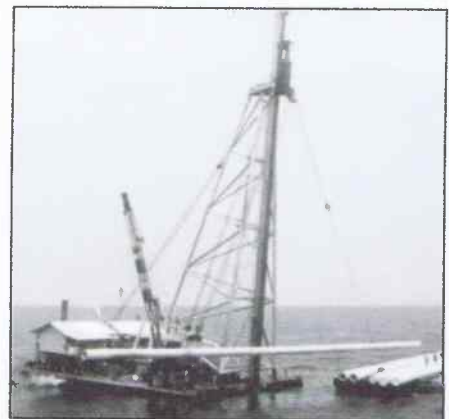
Pile driving barge Rotterdam handling a 36in prestressed concrete pile in Lake Maracaibo in the 1950s.
